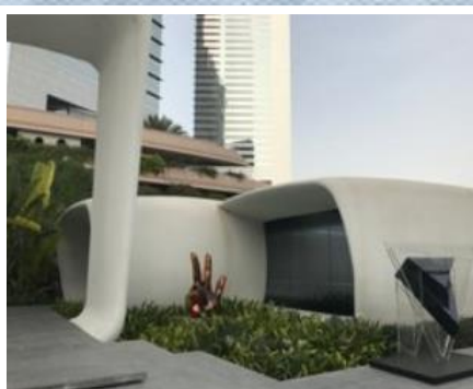
The 3D Printed Office of the Future, Dubai, UAE
